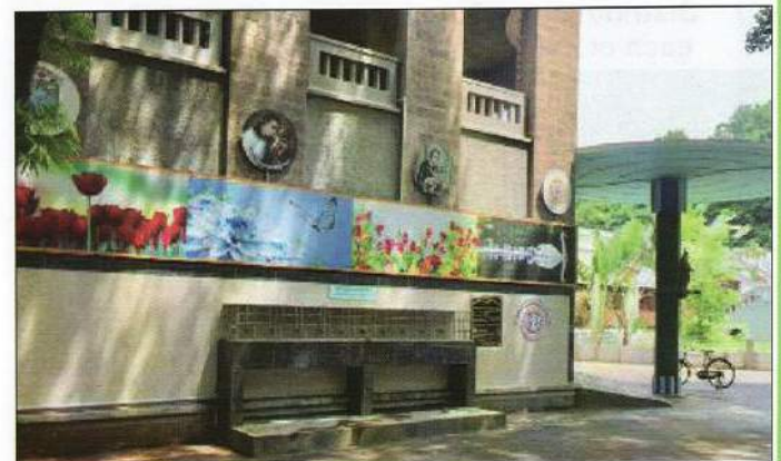
ALCAA installed two water plants for students
